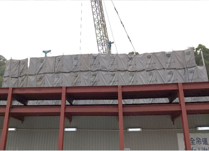
Deployment of Noise Barrier
