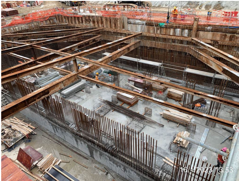
RC Structure for Pumping Station in progress
