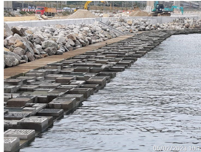
General View of ES2(E)
