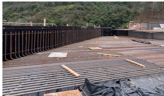
Rebar fixing of base slab of service reservoir
