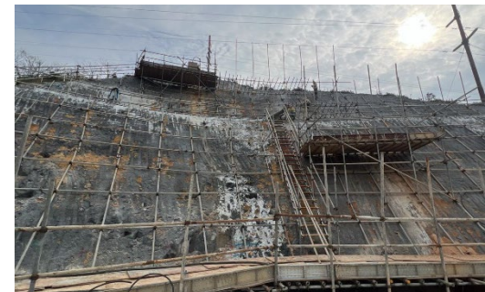
Soil Nail Works
