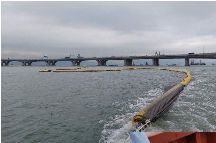
Maintenance of perimeter silt curtain
