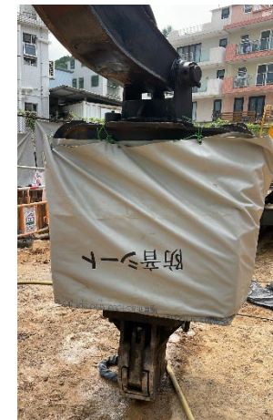
Noise mitigation measures on sheet piling works
