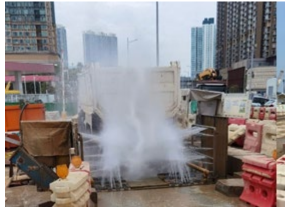
Wheel washing bay with high pressure jet
